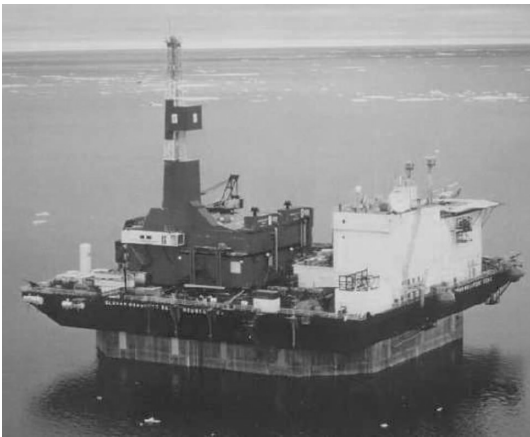
Fig. 3. Concrete Island Drilling System (CIDS) platform constructed with precast and prestressed concrete elements designed to withstand the severe ice-floe pressures of the Arctic. The CIDS platform replaces the building of gravel islands, which cost approximately $100 million to construct, whether oil was found or not. In contrast, the Concrete Island Drilling System cost only $75 million to construct and has been reused for the past 20 years to explore numerous locations along the north Alaskan coastline in the Beaufort Sea without showing any deterioration in the hull. In addition, it leaves no footprint on the seabed. The CIDS is presently operating along the east coast of Russia.
