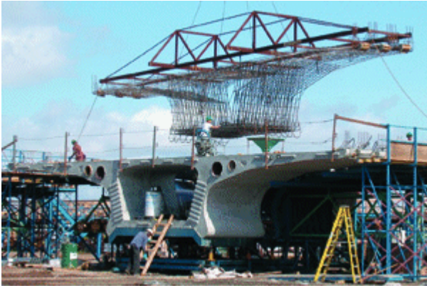
Fig. 3 Match casting, where each new segment is cast against the previously completed one to ensure that all the pieces fit together properly. The curved shape of segments was one of the bridge's aesthetic features.
