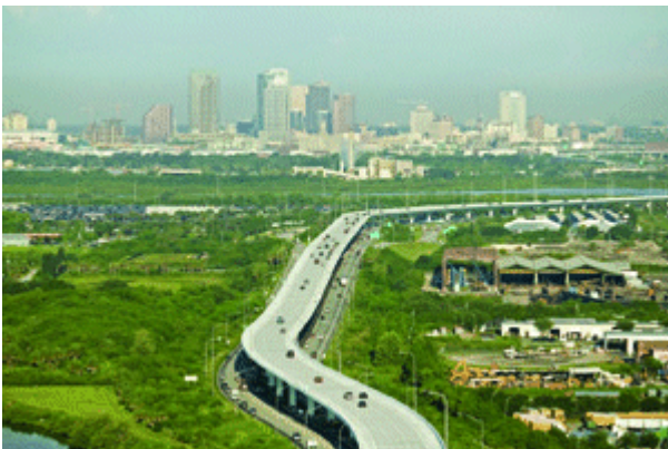
Fig. 1 Elevated bridge on a 6-ft-wide (1.8-m) pier provides the equivalent of six lanes of peak commuting period capacity.
